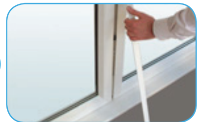
Once locked into position the buttons are used to locate the cover strip
